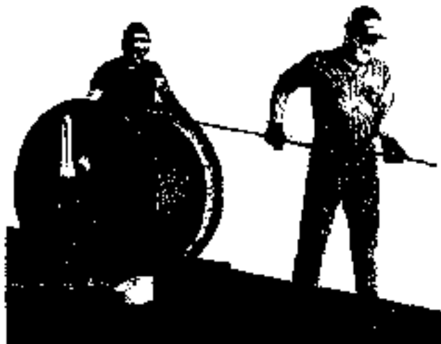
Figure 13. The wire rope reel is mounted on a shaft supported by jacks. This permits the reel to rotate freely, and the rope can be unwound either manually or by a powered mechanism.
