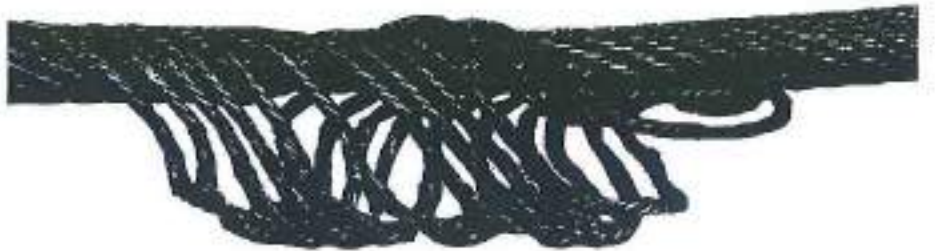
Figure 49. This is a typical bird cage condition.
