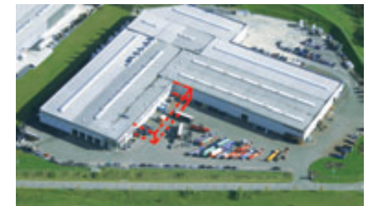
An extra 1,500 m 2 of space has been fitted out at Lentzweiler to reduce the amount of time semi-trailers spend in the production hall.
