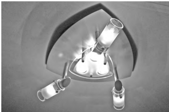
Ceiling light above the middle seating arrangement (depending on the model) can be switched manually directly on the lamp.
