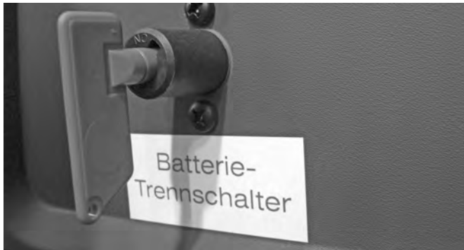
Battery circuit breaker
