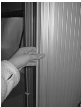
Sliding door in washroom
