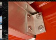
Wilson's aluminum crossbar clips are attached to the main beams and the crossbars using corrosion resistant stainless steel fasteners. A copolymer material is also placed between the aluminum clip and steel beam to insulate the two dissimilar metals. Couple this concept with the insulating
