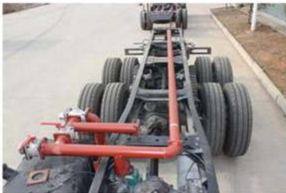
Overlook for pipeline
